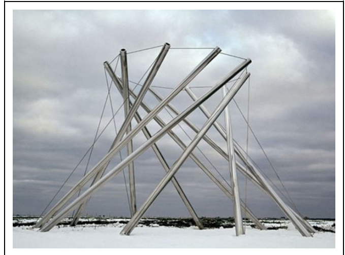
Figure 1. Tensegrity. A structure is stabilized by the balance of a constant tension and by the presence of a discontinuous compression. This organization is self-stabilizing, allowing to manage tension variations with a certain degree of flexibility, transferring the forces applied to the whole structure. The photo shows the sculpture by artist Kenneth Snelson.
